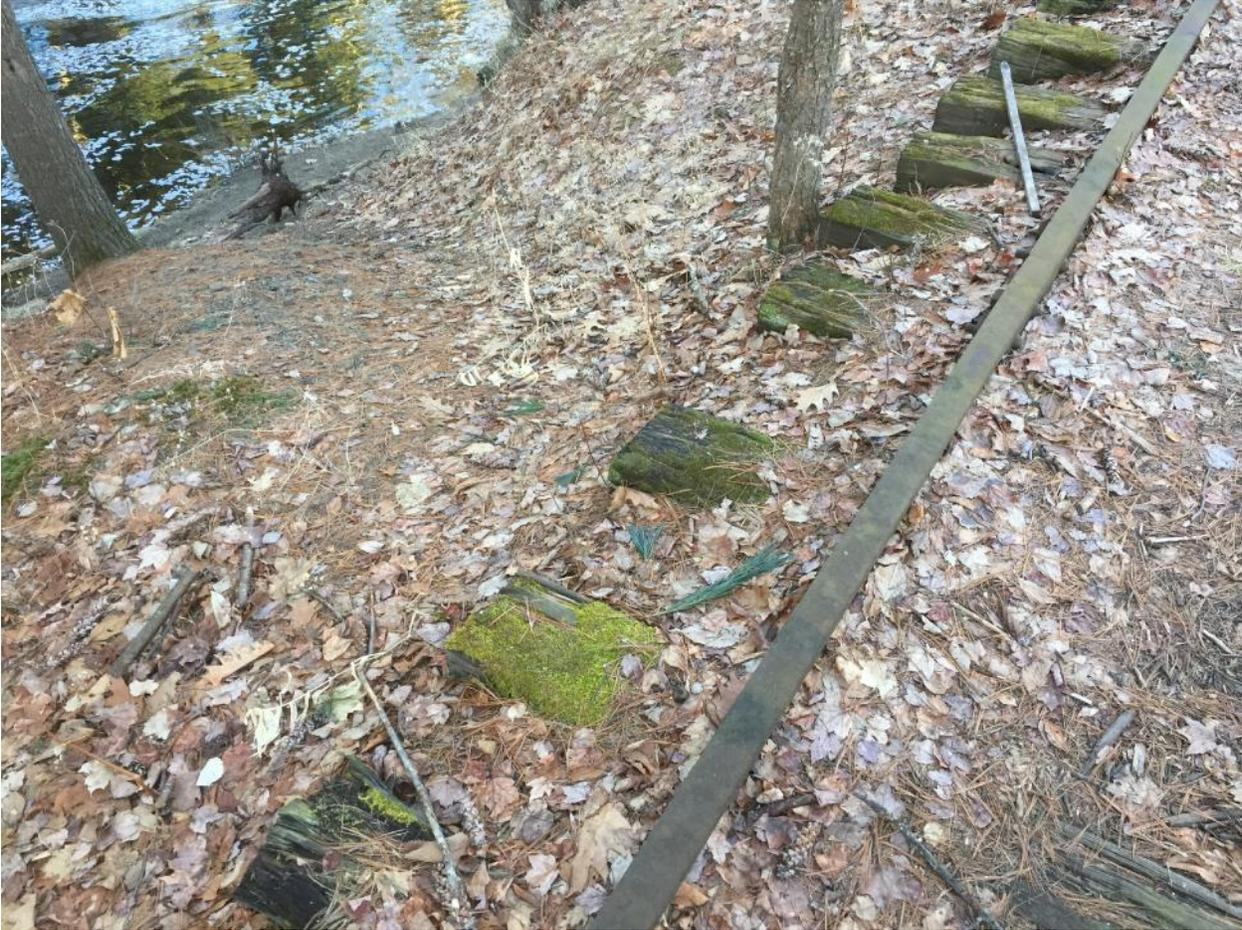
Area 1, Erosional swale leading down to river and undercutting rail bed
